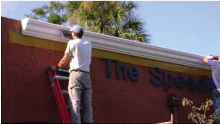
Workers adding and painting crown molding to roof of JSHC.
